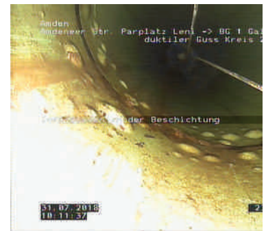
Air Bubbles Below Coating
